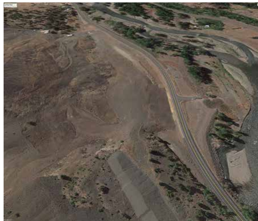
The 2009 landslide included a tremendous volume of soil, as the entire hillside slid over the highway and into the river valley. Photo from Google Earth.
