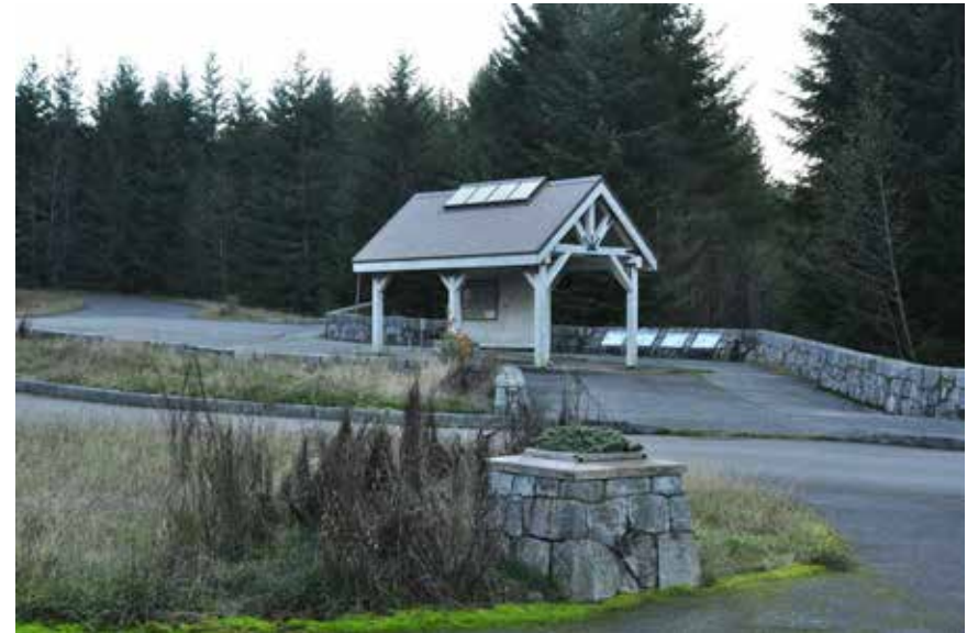
The Mount Rainier Viewpoint is a popular visitor site on the byway, but is also a significant management challenge. Stakeholders would like to see improvements here including restrooms, clearing to open views of Mount Rainier, and interpretive updates.
